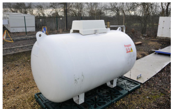
Figure 89 LPG tank
