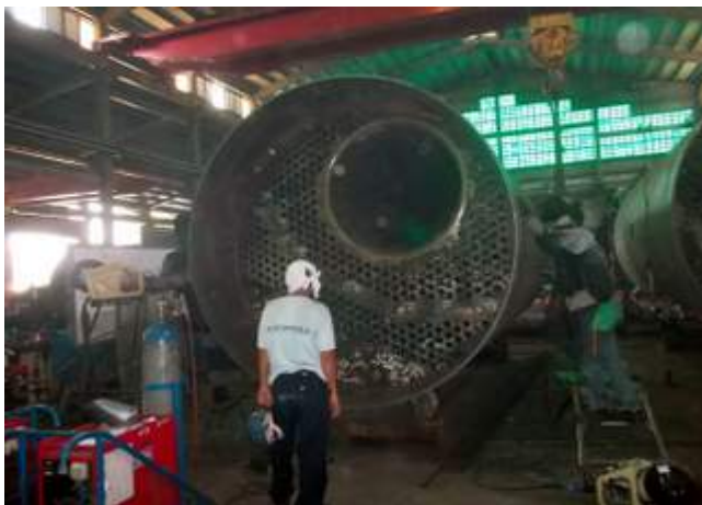
Figure 70 Boiler manufacturing-combustion chamber and tube sheet (Courtesy of Enertech-Philippines)
