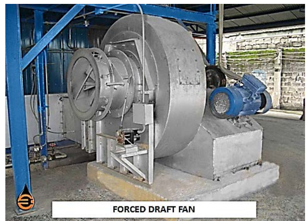
Figure 45 Forced draught fan-(Courtesy of Eneritech –Philippines)
